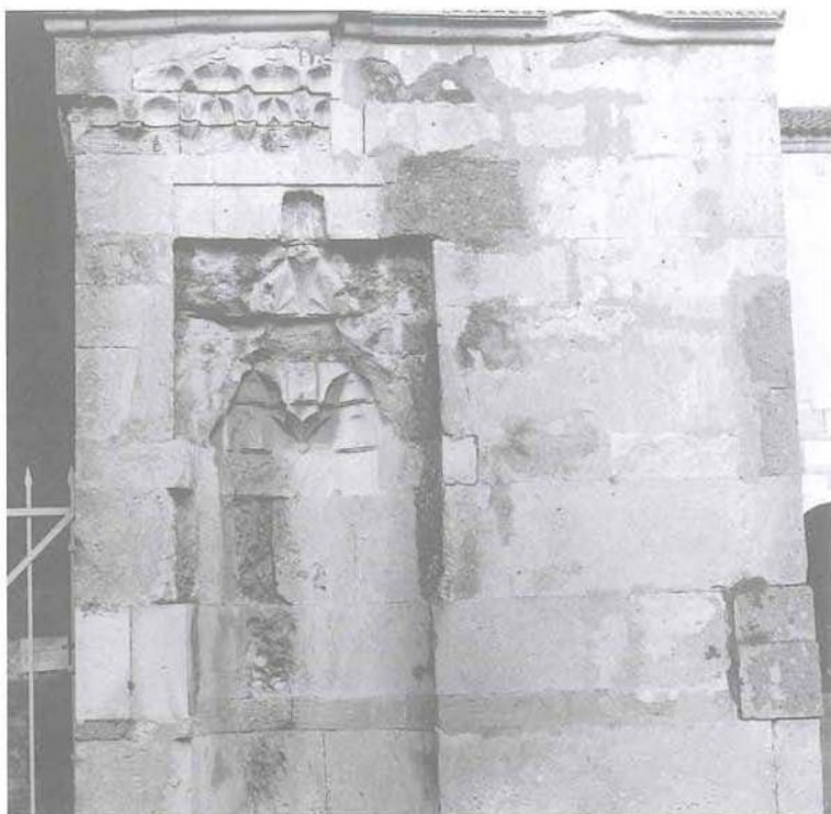
48 West porch of Hagia Sophia. Complex muqarnas work is visible in the niche and below the cornice
